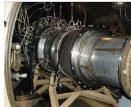
COMBUSTOR ▪ Definition of design configuration ▪ Combustor tests at C5-2 test cell
